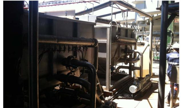
The floated solids are collected at the tank surface by a chain scrapper which sweep the scum towards an outlet hopper to thicken up to 4 – 5% DS content before flowing to the sludge treatment. The solids that sediment in the tank are extracted through a screw installed at the tank bottom connected to an automatic purge valve. The sludge separated in the DAF is calculated as 300 m<sup>3</sup>/day further dewatered in a centrifuge decanter.
