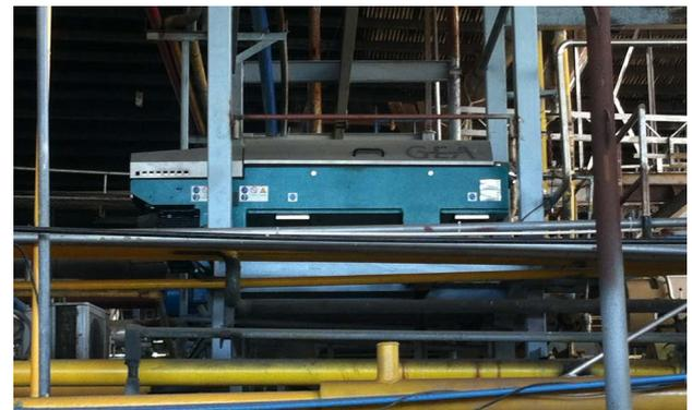
SIGMADAF scope of supply included the DAF equipment, wastewater lifting pumps pipes and valves, sludge pump, sludge decanter, the chemicals preparation and dosing, mixers, instrumentation for level, flow, pH, pneumatic panel, electrical switch panel (MCC) and control panel with PLC, cabling, transportation, spare parts, supervision on site during erection-installation, start-up and training, as a turn-key complete scope.
