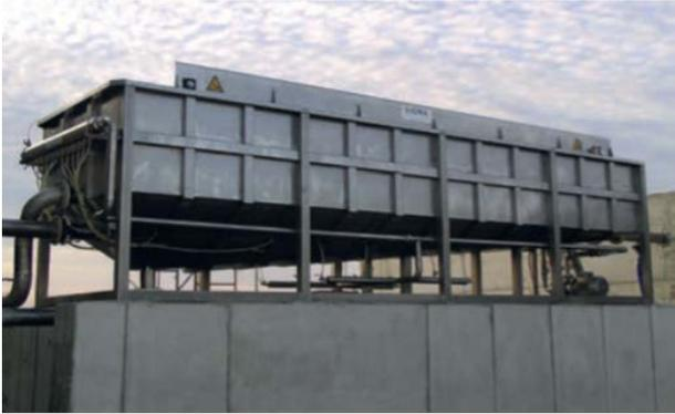
The FPAC incorporates an aeration system (pump – saturator – valves) to generate micro-bubbles (30 to 50-micron range) to increase efficiency, as smaller bubbles easily adhere to equal-sized or larger solid particles, enhancing the overall flotation effectiveness of the system.
